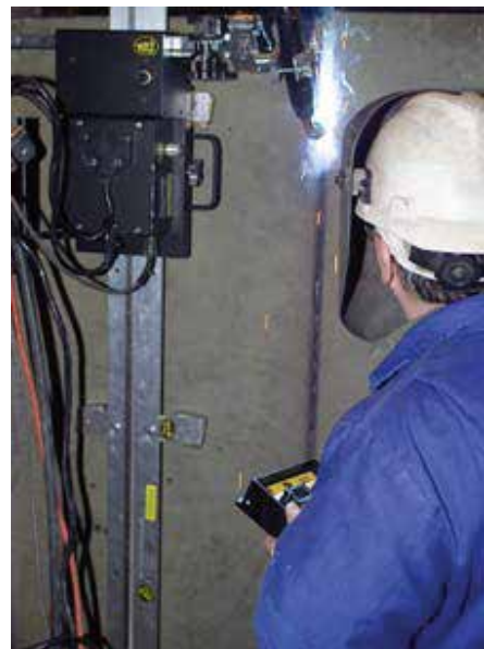
Shown Above - Vertical Weld
