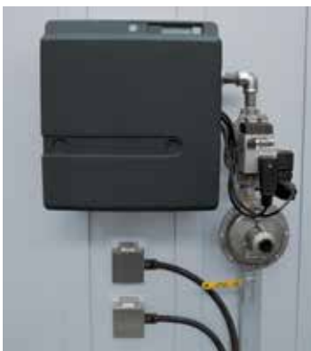
Compact burners for standard models up to NB 600
